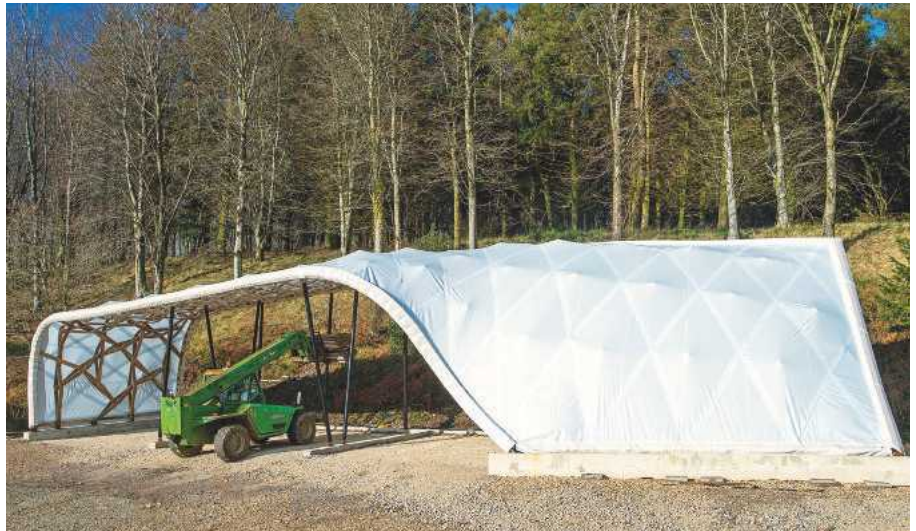
...and is ready for its waterproof cover
